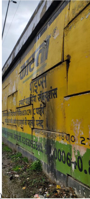
Figure 2 (Continued) Photographs depicting bulging of RE wall at km 102+570
