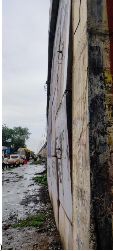
Figure 2 (Continued) Photographs depicting bulging of RE wall at km 102+570
