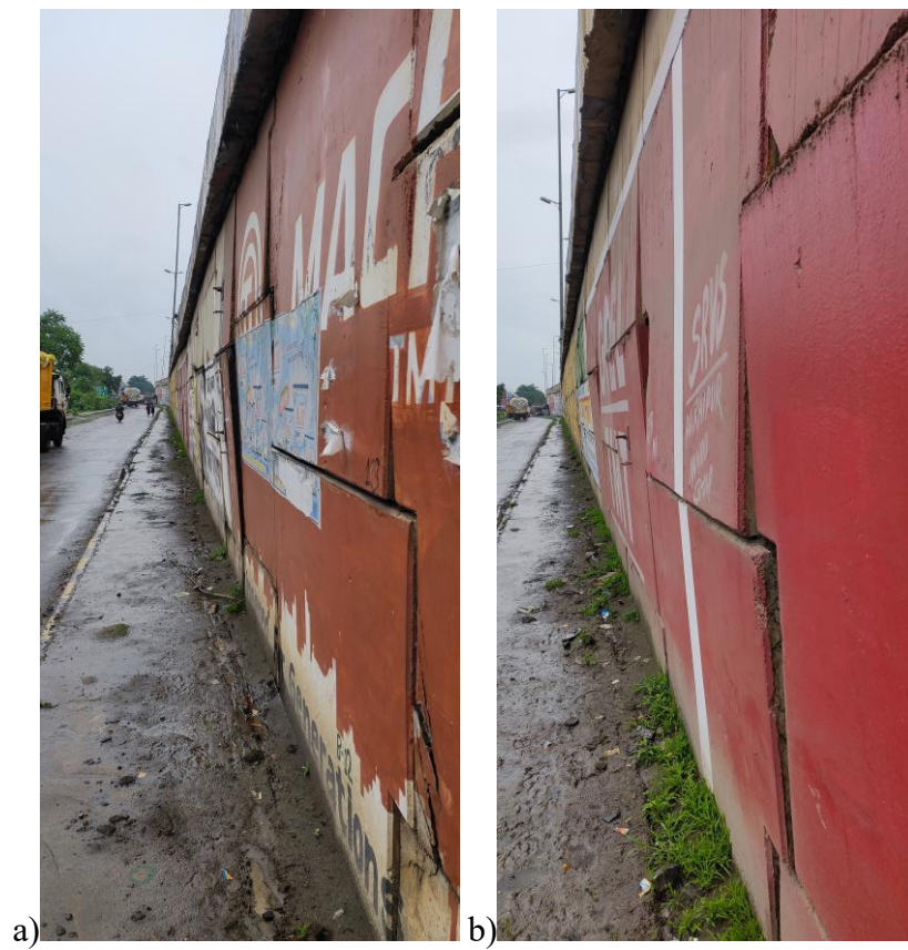
Figure 2 Photographs depicting bulging of RE wall at km 102+570
