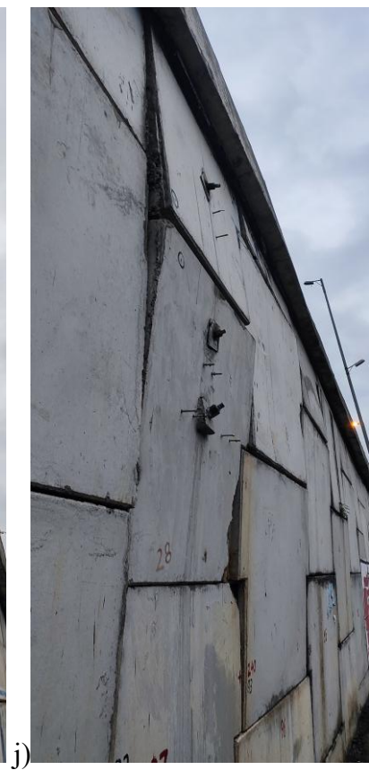
Figure 3 (continued) Photographs depicting bulging of RE wall at km 96+426
