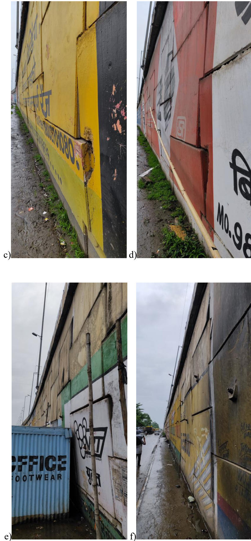
Figure 2 (Continued) Photographs depicting bulging of RE wall at km 102+570
