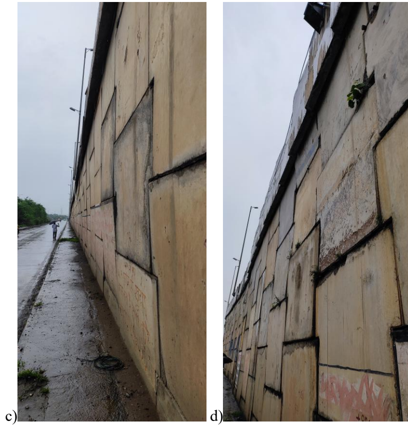
Figure 1 Photographs depicting bulging of RE wall at km 106+224
