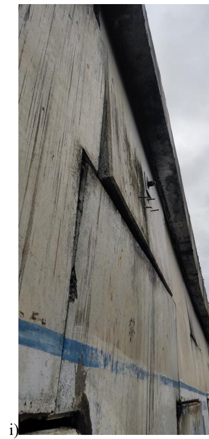
Figure 3 (continued) Photographs depicting bulging of RE wall at km 96+426
