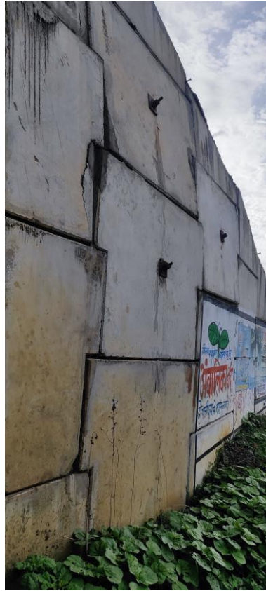
Figure 4 Photographs depicting bulging of RE wall at km 91+816
