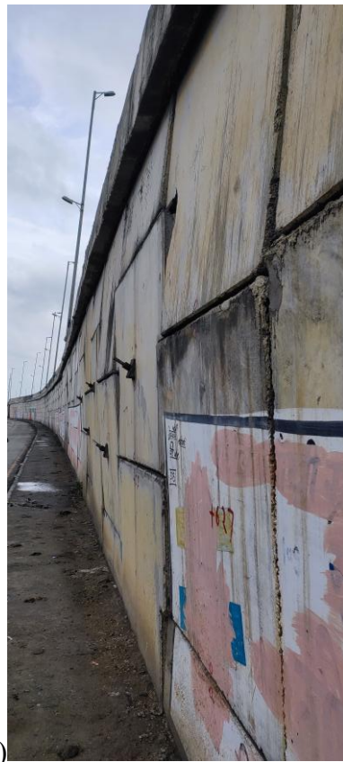
Figure 3 Photographs depicting bulging of RE wall at km 96+426
