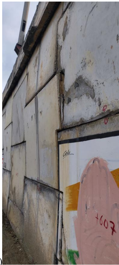
Figure 3 Photographs depicting bulging of RE wall at km 96+426
